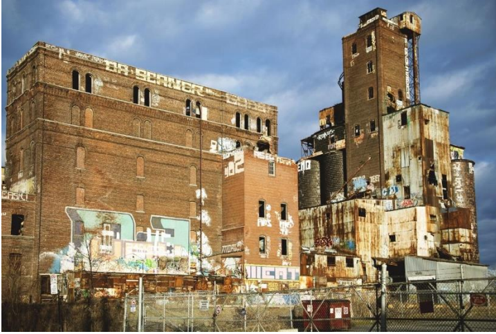
Photo 11: Canada Malting Plant, Montréal, 2010.
