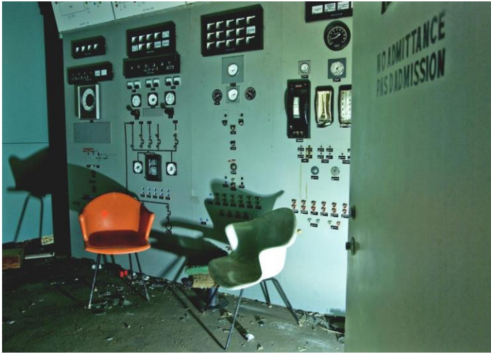
Photo 17: Bunker militaire, Saint-Raymond-de-Portneuf, Québec, 2010.
