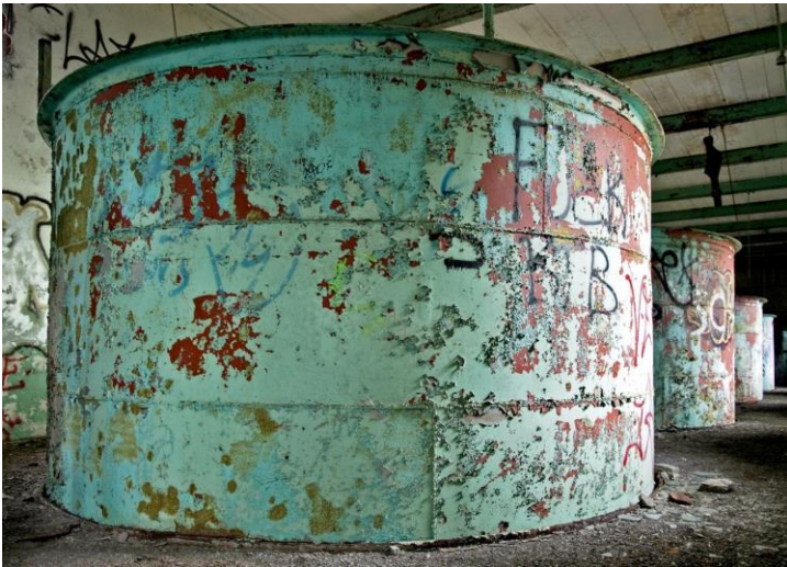
Photo 12: Canada Malting Plant, Montréal, 2010.
